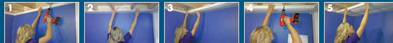
2) Insert the first panel into the wall trim
